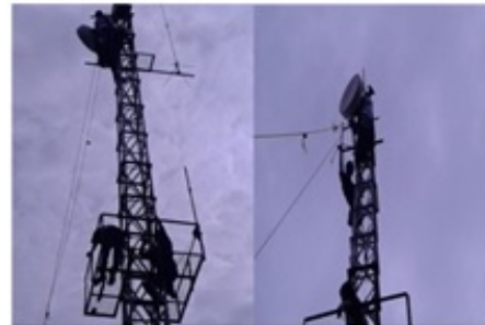
Figure 3. Tower at site Pakuhaji
