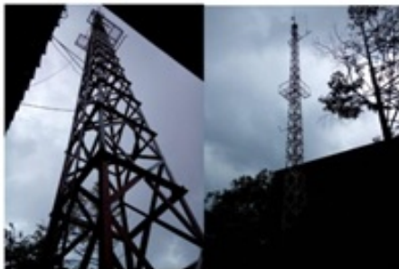
Figure 2. Tower at site Polban
